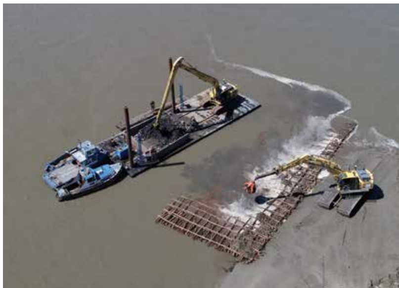
Img.58 Placing fascine mattress.
