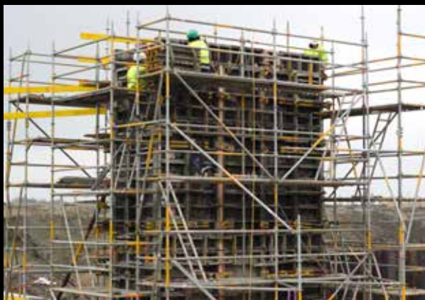
Img. 35 Concrete works.
