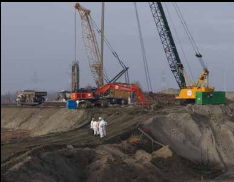
Img.27 Installing piling sheets in CB wall.
