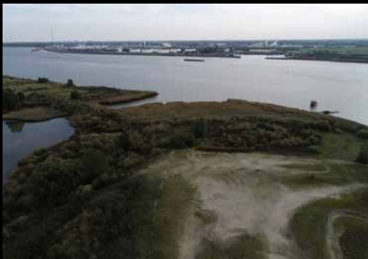
Img.14 General progress, October 2019.
