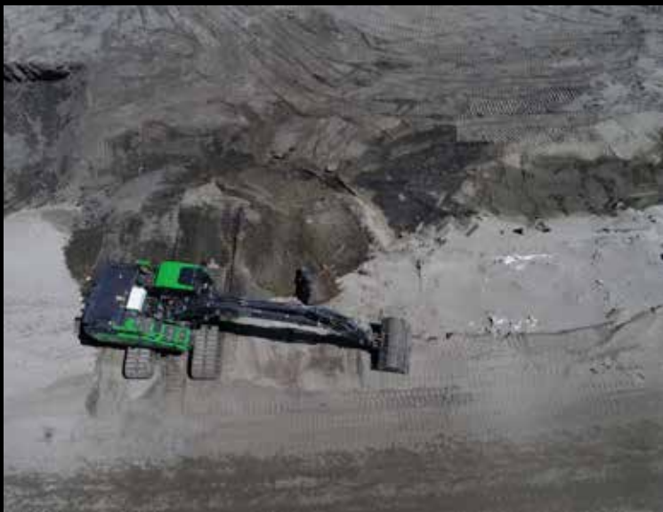
Img.28 Remediation Zone 4.
