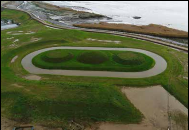
Img. 26 General progress, November 2021.
