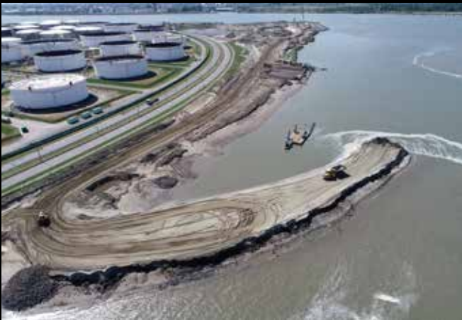
Img. 61 Creating ground dike.
