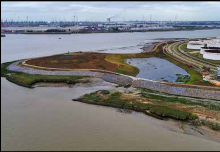
Img. 24 General progress, September 2021.
