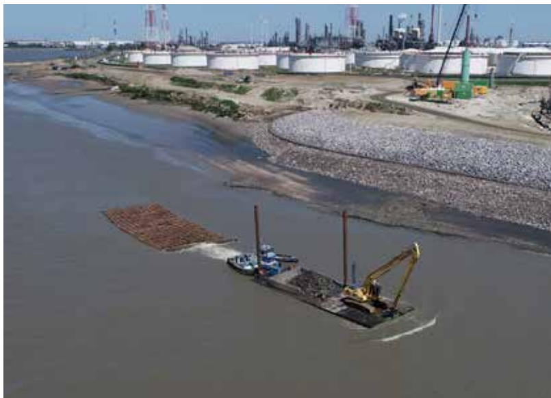
Img.57 Transport fascine mattress.
