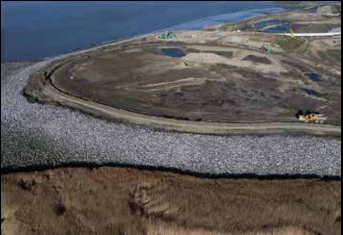
Img. 18 General progress, November 2020.
