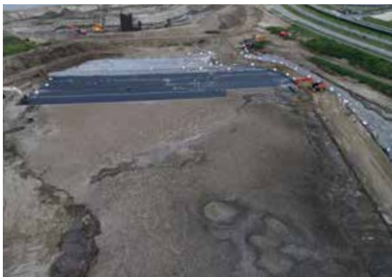
Img. 43 Cover with HDPE liner and geosynthetic clay liners.
