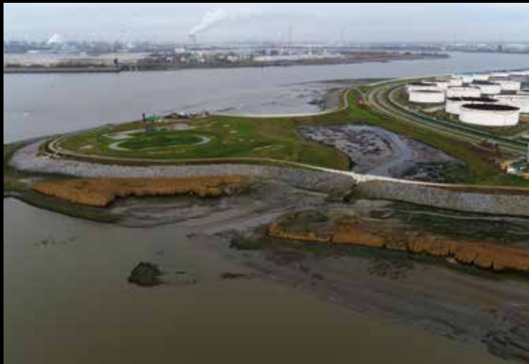
Img. 25 General progress, November 2021.
