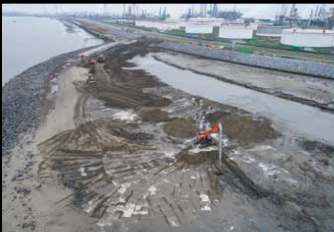
Img.74 Elimination of over-height (infill between Scheldt and crib dike).
