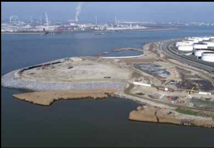
Img. 19 General progress, March 2021.
