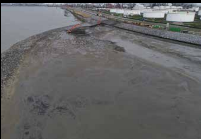
Img.75 Elimination of over-height (infill between Scheldt and crib dike).
