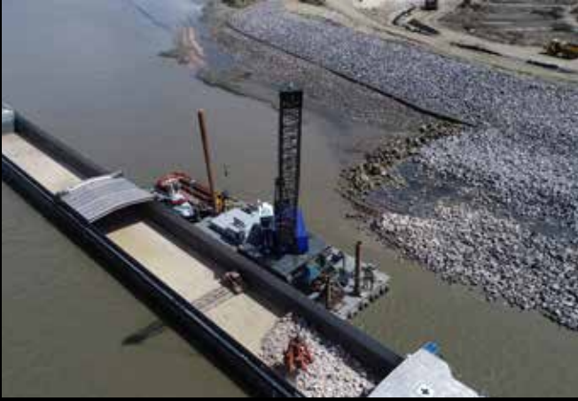
Img.72 Depositing crushed stone.
