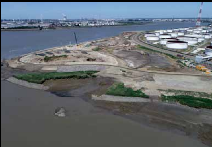
Img. 16 General progress, May 2020.
