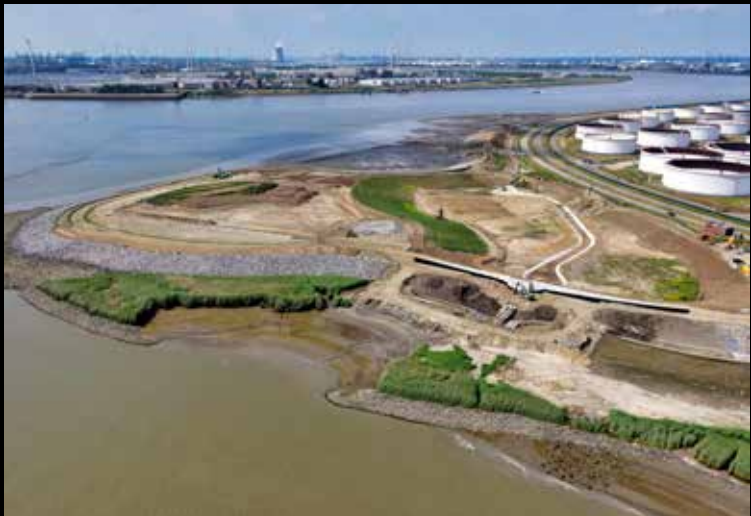
Img. 20 General progress, June 2021.
