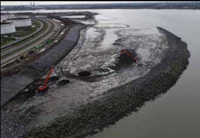
Img.73 Elimination of over-height (infill between Scheldt and crib dike).
