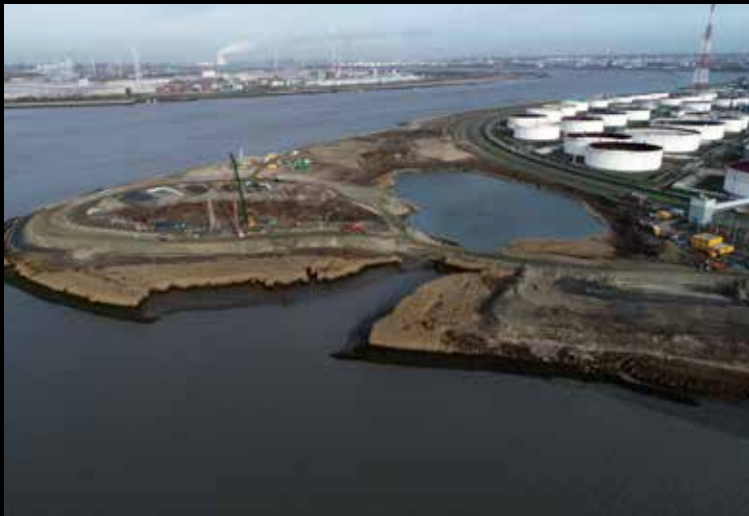
Img. 13 General progress, January 2020.
