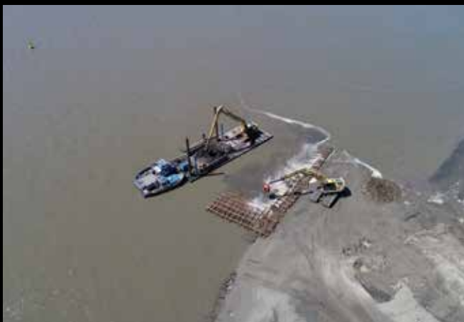
Img.70 Placing and ballasting fascine mattresses.
