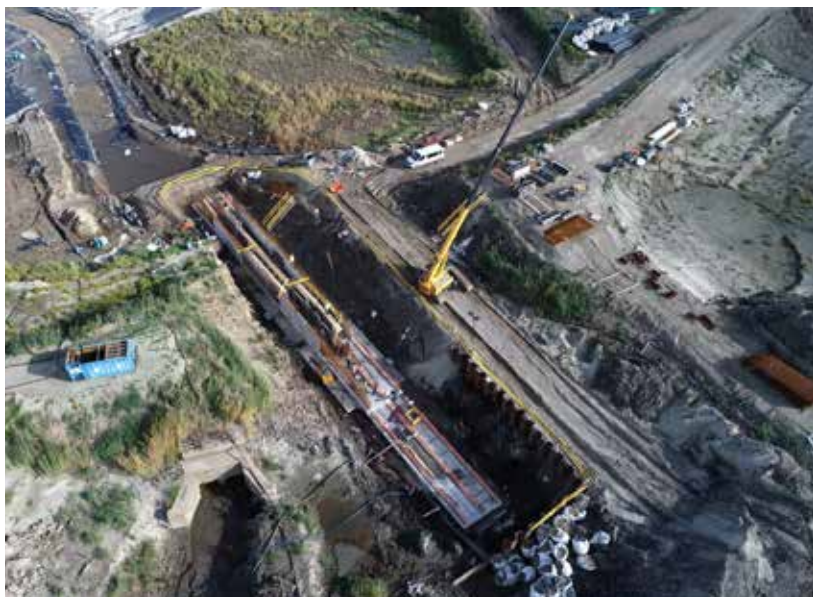
Img.55 Civil retaining wall UW.
