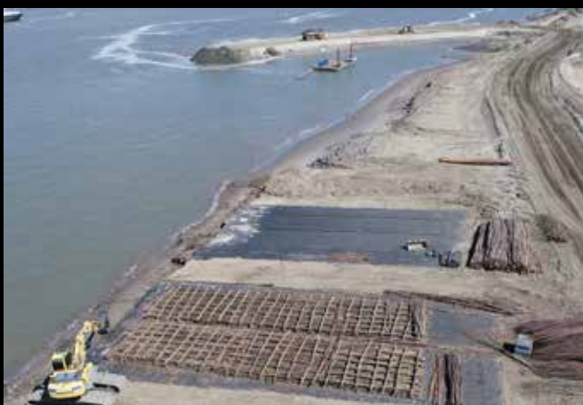
Img.67 Prefab zone fascine mattresses.
