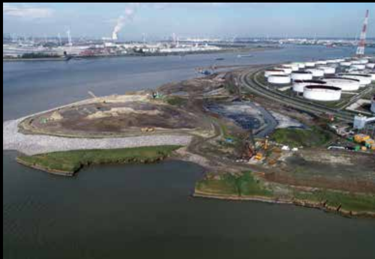
Img. 17 General progress, September 2020.
