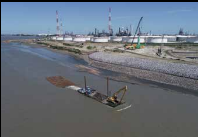
Img.68 Sailing in fascine mattresses.
