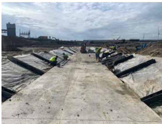
Img.48 Side of the channel.
