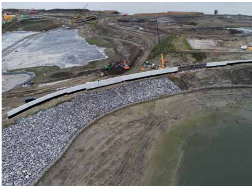
Img.50 Civil retaining wall north.
