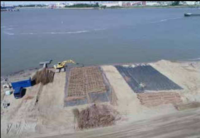
Img. 65 Prefab zone fascine mattresses.
