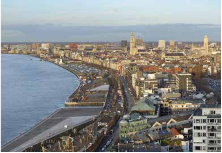
Img.07 Example of a Sigmaplan project. Works on the Scheldt quays at Sint-Andries and Het Zuid.
