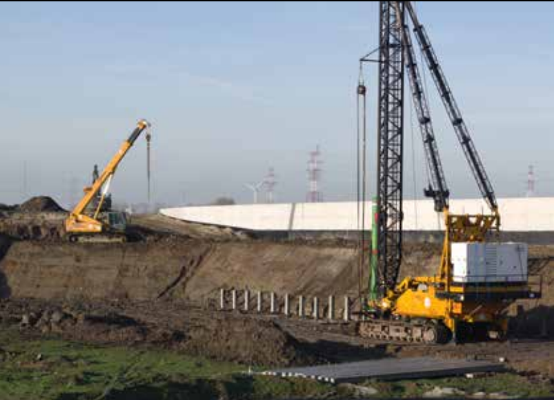
Img.33 Placing concrete piles.
