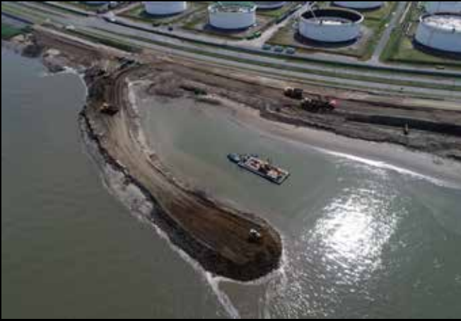
Img. 60 Creating ground dike.
