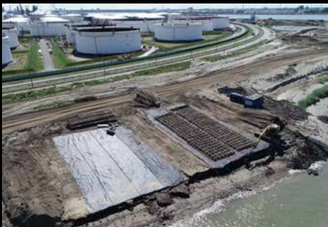
Img.66 Prefab zone fascine mattresses.
