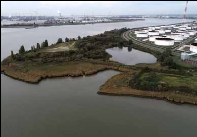
Img. 12 General progress, October 2019.
