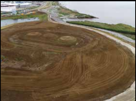
Img.21 Detailed progress, June 2021.
