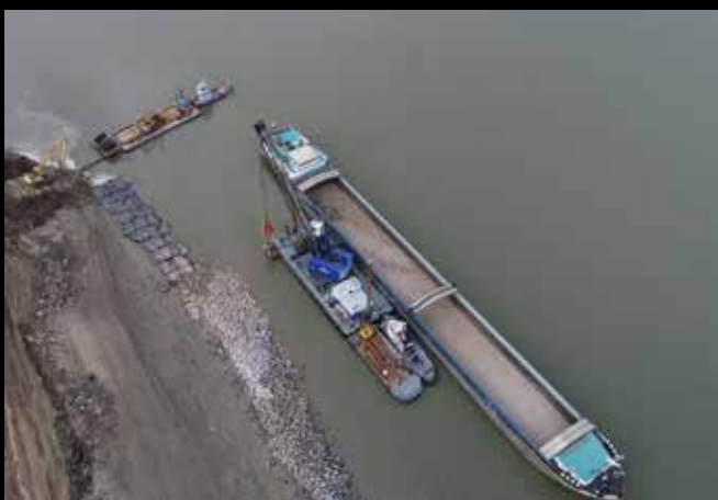
Img.71 Depositing crushed stone.
