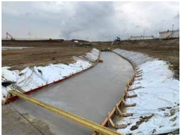
Img. 45 Excavation of the channel.
