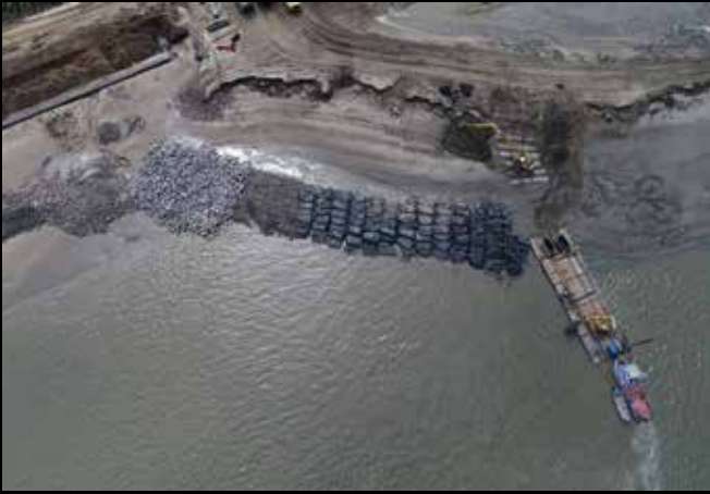
Img. 64 Placing geotextile elements after profiling dike.
