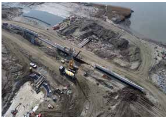
Img.51 Civil retaining wall south.
