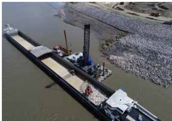
Img.59 Crane ship.
