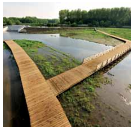
Figure 2.5. The walkway in Bergenmeersen with bridge over the eastern stream arm
