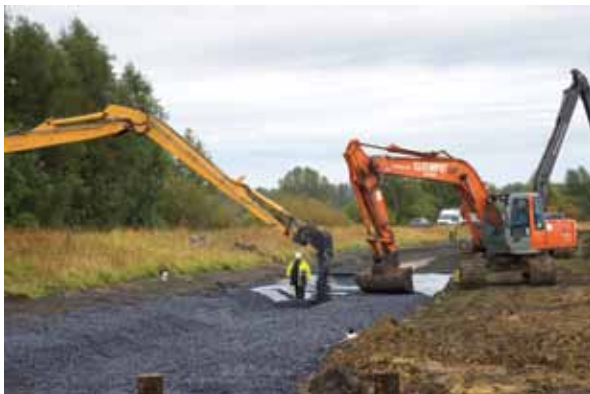
Figure 7.12. Construction of dissipation channel with open stone asphalt
