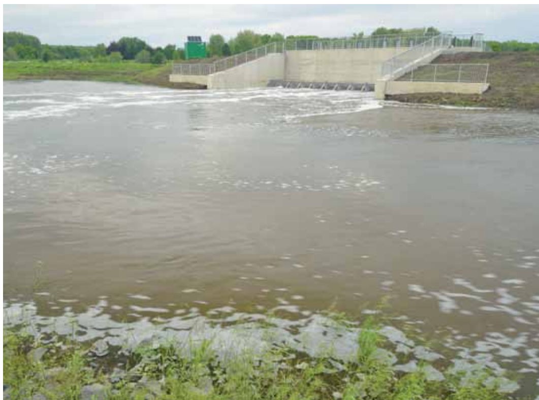
Figure 7.14. A completed FCA-CRT
