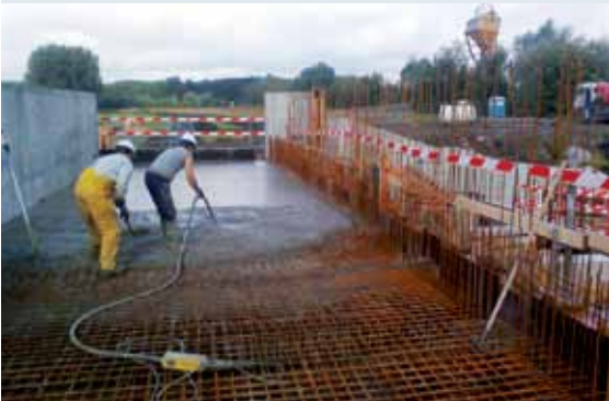
Figure 7.6. Floor slab and sheet piles against seepage
