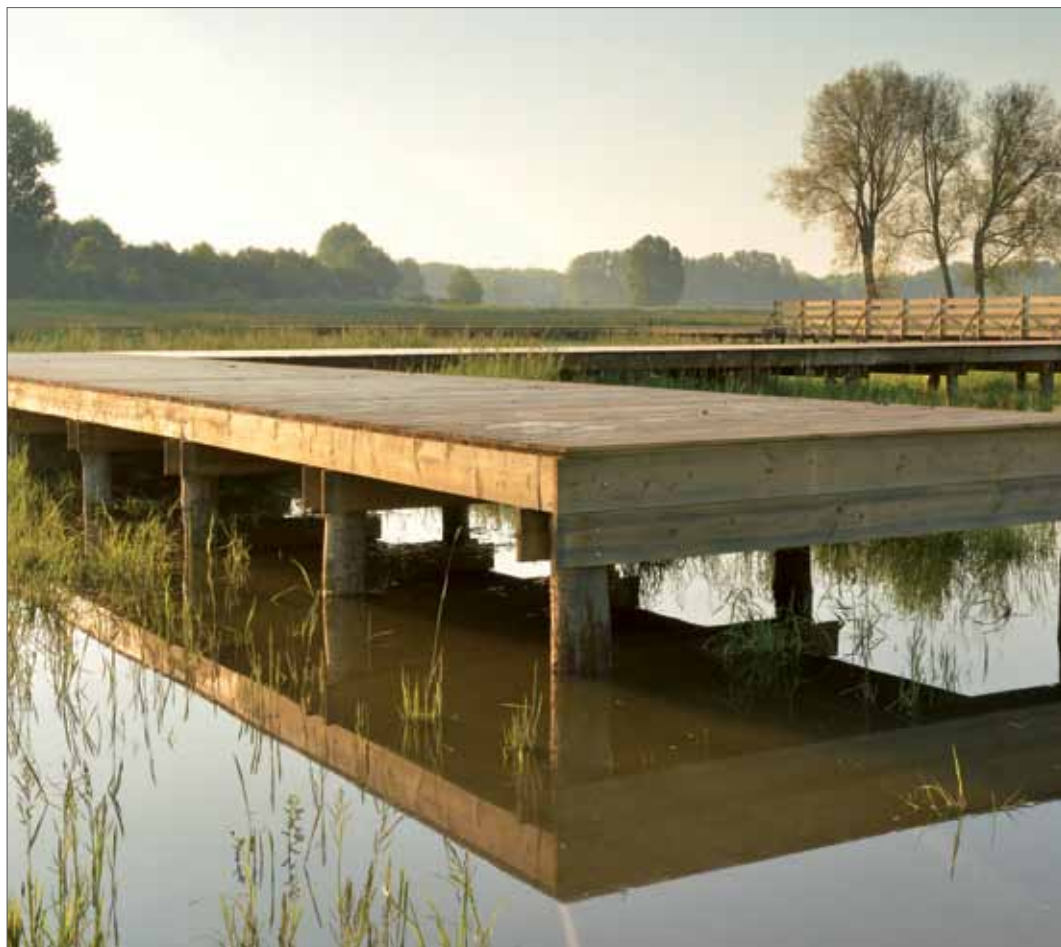
Figure 3.9. Walkway in Bergenmeersen
