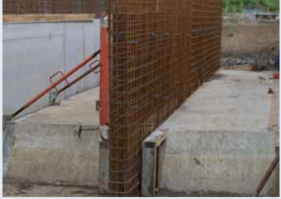
Figure 7.5. Formwork and reinforcement of the walls
