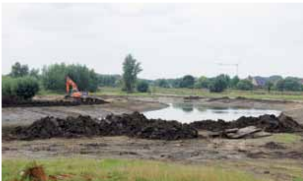
Figure 73. Earthworks: end of excavating the channel source
